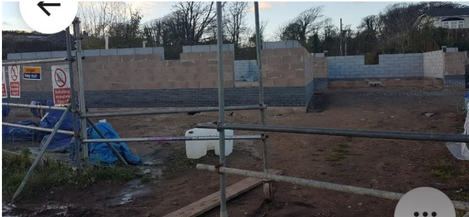
Appendix 4: Photograph dated 7 November 2016, showing the dwelling's external walls under construction at low level, Egremont
